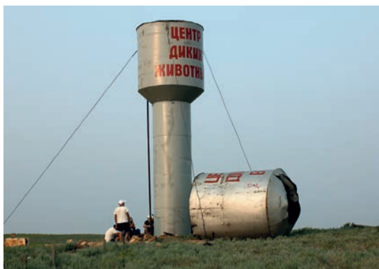
Figure 26. Installation of the Rozhnovski water tower in the Yashkul Captive Breeding Station (Photo by Yu.N. Arylov).
